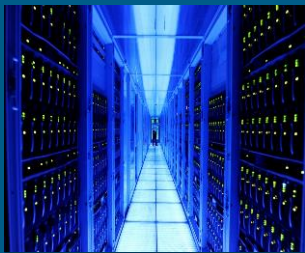
On-Site Data Center
